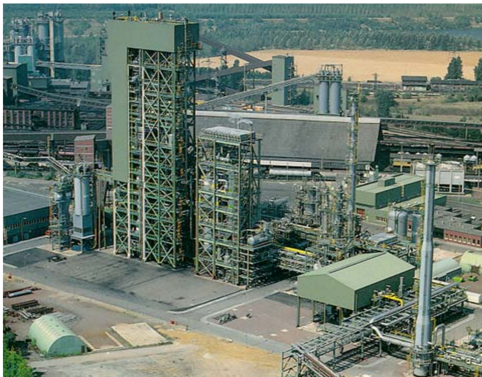
Fig. 5: HTW Demonstration Plant Berrenrath, Germany Production Rates: 300 t/d Methanol, Total Operating Hours: 67,000h [7]
